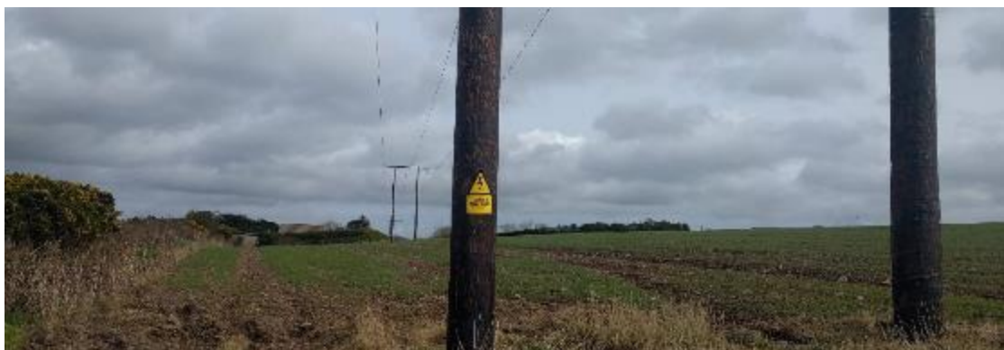
Photograph 5 Northern section of the 110kv powerline wayleave corridor
