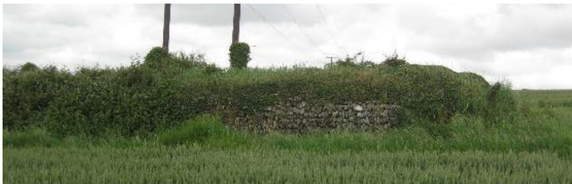
Photograph 6 Example of existing sod and stone ditch on site
